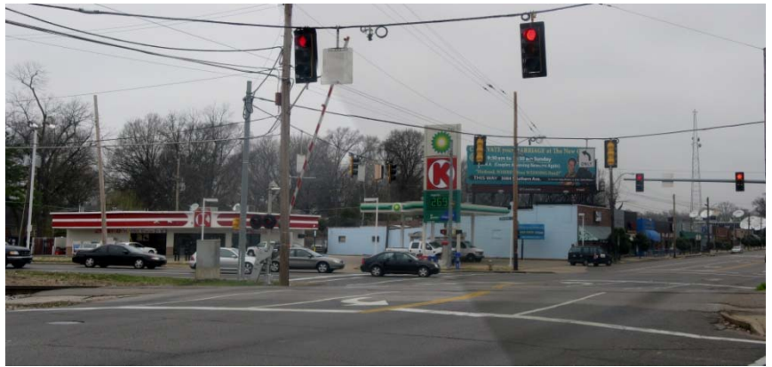
Existing Conditions at the intersection of Highland St. and Southern Ave.
