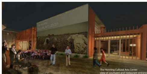
The Henning Cultural Arts Center view of courtyard and restaurant entrance Henning Cultural Arts Center Courtyard
